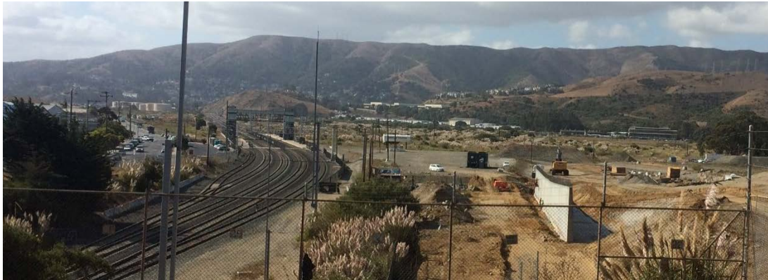
Figure 38 Caltrain Right-of-Way Facing South from Blanken Avenue 22
